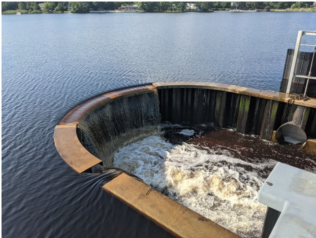
Figure 1. Primary Spillway operating at normal pool level. Lake elevation \pm 2 inches above low-flow weirs
