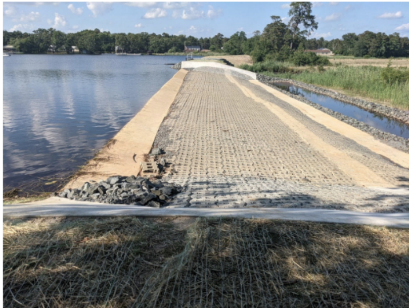
Figure 2. Secondary Spillway operating at normal pool level. Lake elevation 2" below upstream concrete apron
