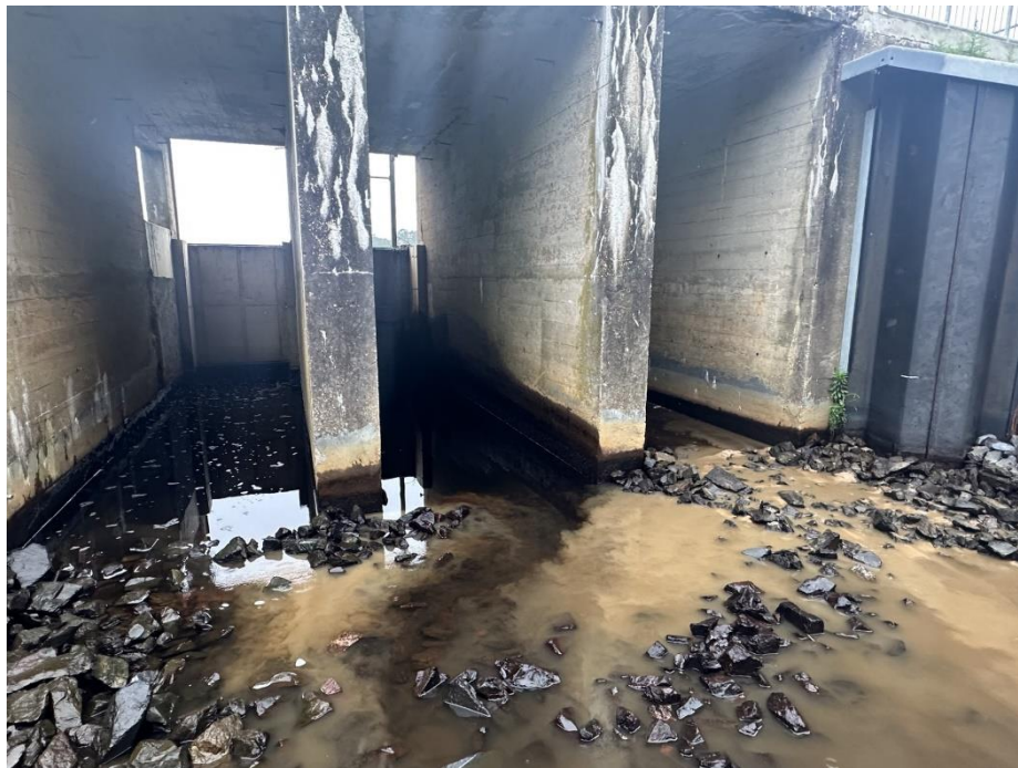
Photo 6: Boils with silt infiltration at downstream end of Northern Auxiliary Spillway and south interior wall after wading and probing.
