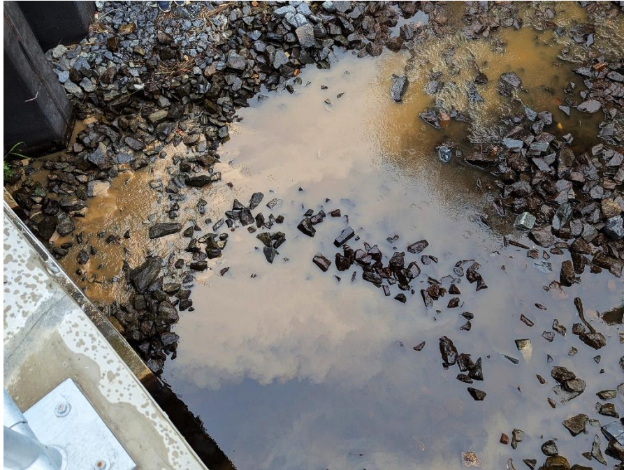
Photo 5: Initial view of silt plumes forming at the downstream end, emanating from near the boils in Photo 3.
