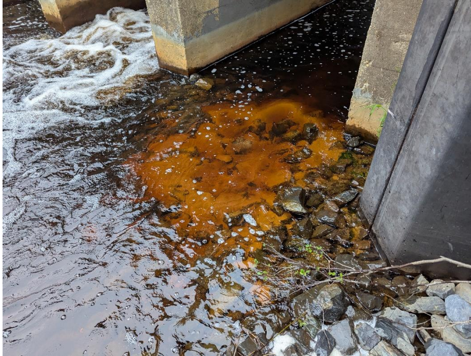
Photo 3: Close-up of boils at downstream end of Northern Auxiliary Spillway before closing the sluice gate.
