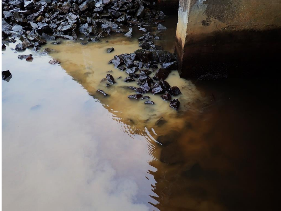
Photo 7: Detail view of the boil and silt plume at the south wall of Cell 2.
