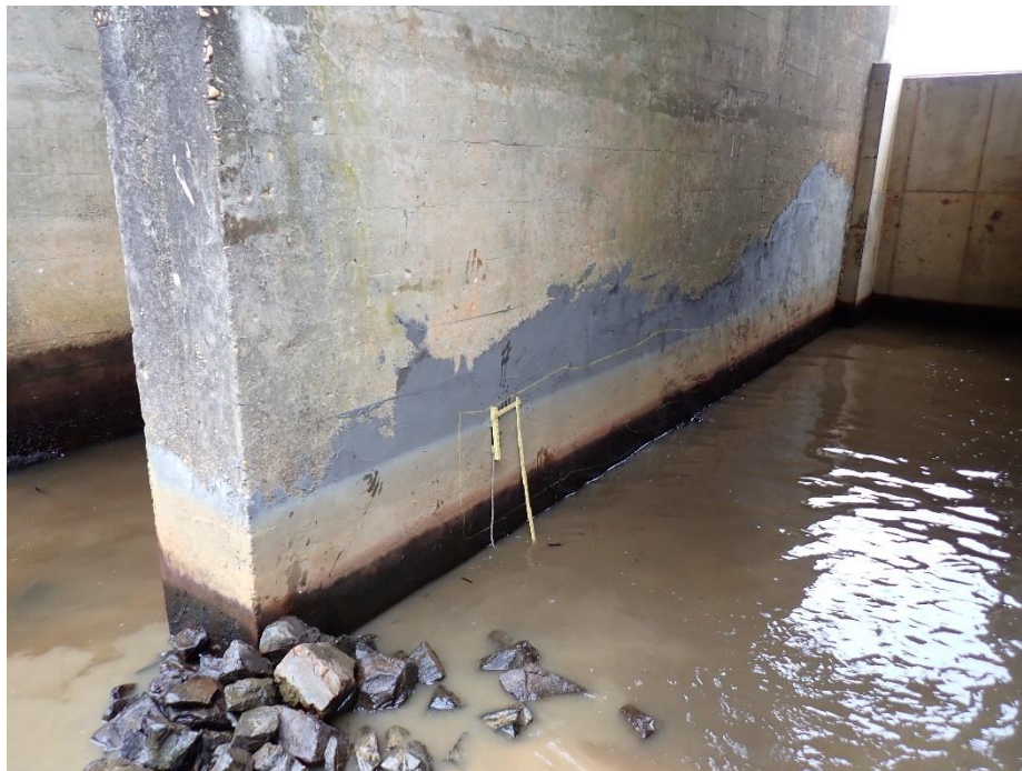
Photo 10: Cell 2, north face of south wall. Typical hollow soundings of rehabilitated concrete.
