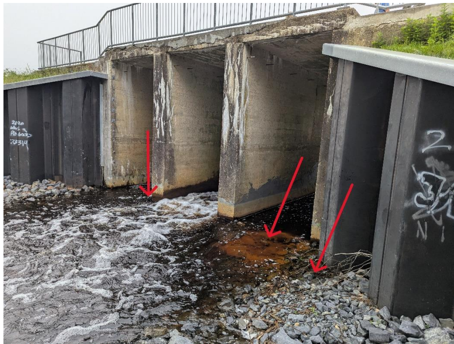
Photo 2: General view, lake side dam structure, east (downstream) face, prior to closing the sluice gate. Area of boils shown by arrows. Note, left location not observed until after wading and probing.
